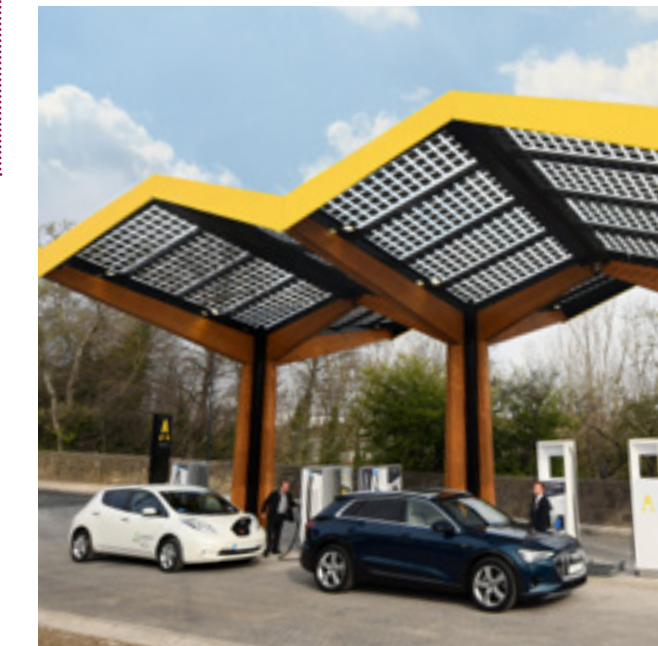
Fastned first rapid charging station, Sunderland
