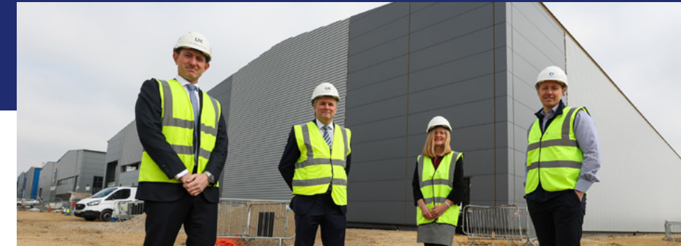
Construction has started on a new £4.5m speculative development on the Tyne Tunnel Trading Estate which has received GBF funding.
