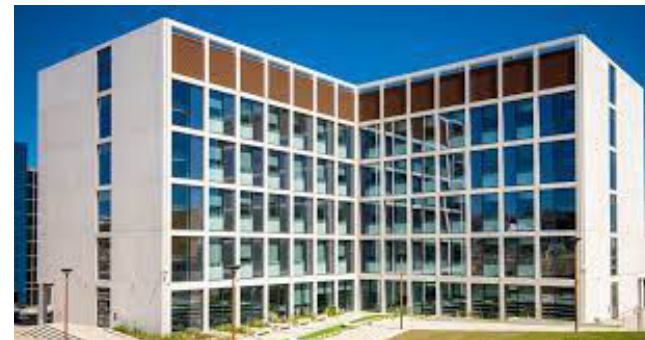
The Biosphere building situated on Newcastle Helix. The North East LEP is providing funding for Newcastle City Council to develop a business case for the creation of a Biosphere 2.
