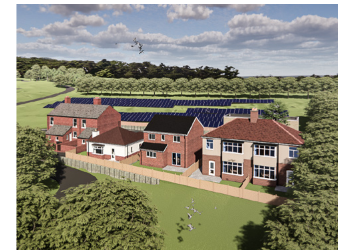
InTEGReL Customer Energy Village – research facility consisting of retro houses constructed to enable real time testing of new technologies and products
