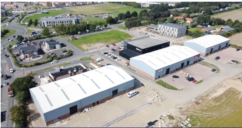
First Commercial Property Investment Fund (CIPF) supported scheme – new units at Thinford, County Durham
