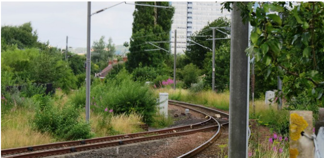
Bensham: Electric power lines over a freight-only line track curving from the Team Valley towards Metrocentre
