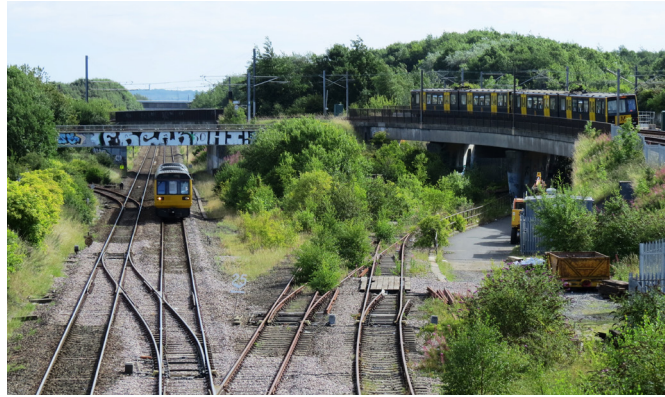
Pelaw: The mothballed Leamside line (centre right) meets busy Metro and rail routes from South Shields and Sunderland
