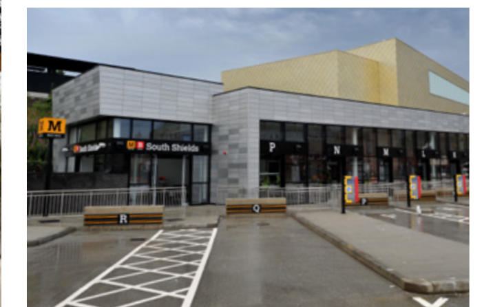
South Shields Interchange
