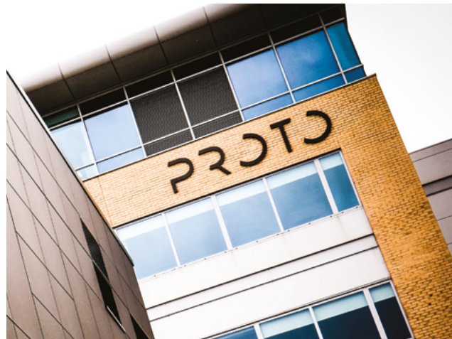
PROTO in Gateshead – an emerging technology centre home to some of the region's most innovative businesses
