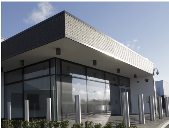
Cobalt Park data centre, North Tyneside
