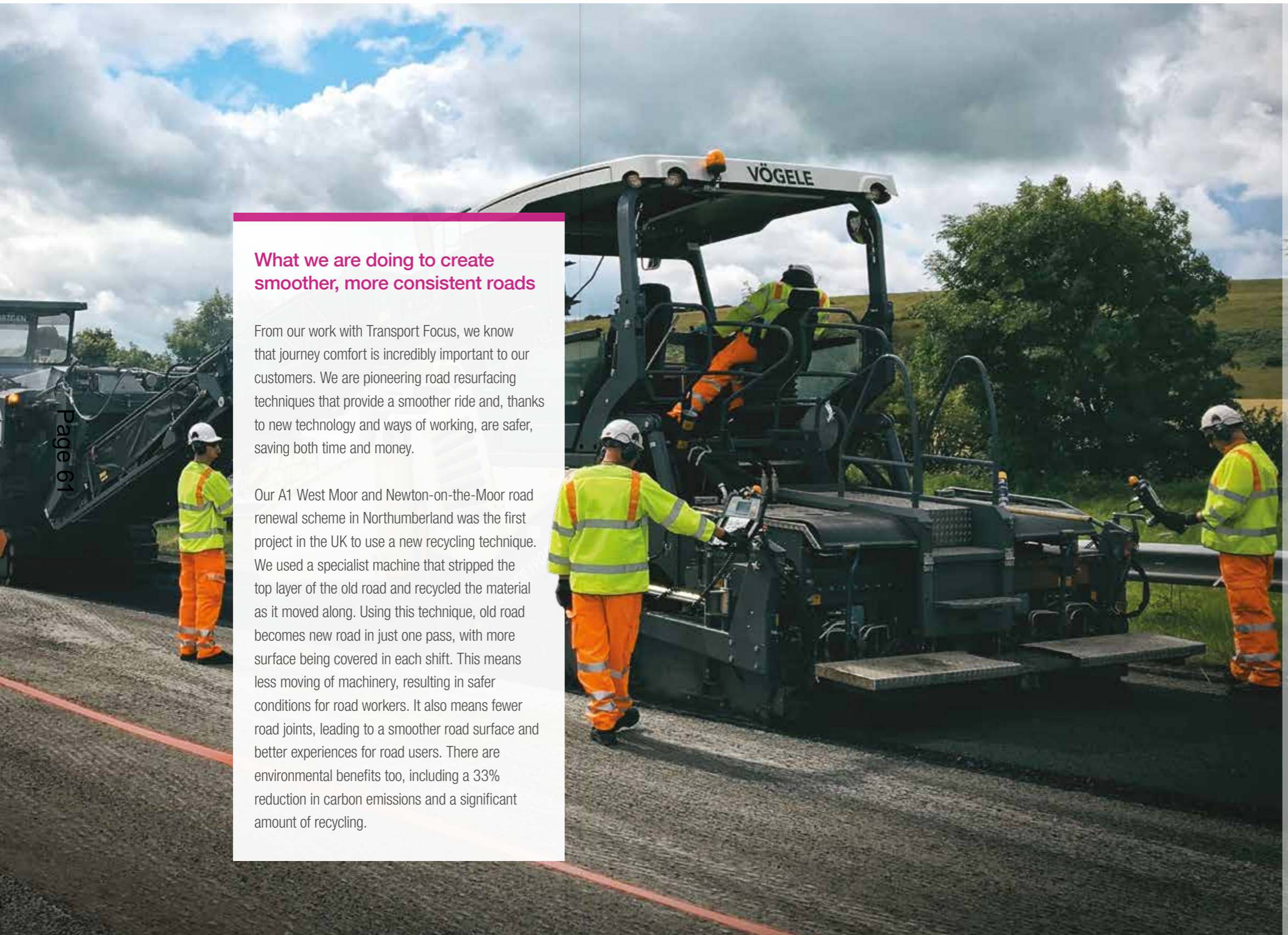
Cold pave technology: Image courtesy of A-one+
