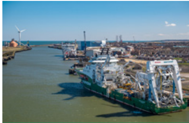
Port of Blyth in Northumberland – the second largest port in the region by turnover and a nationally significant offshore energy hub
