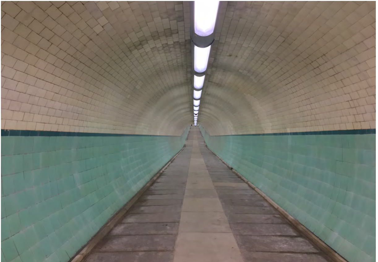
The cleaning of the pedestrian tunnels is nearing completion in preparation for the reopening of the tunnels.
