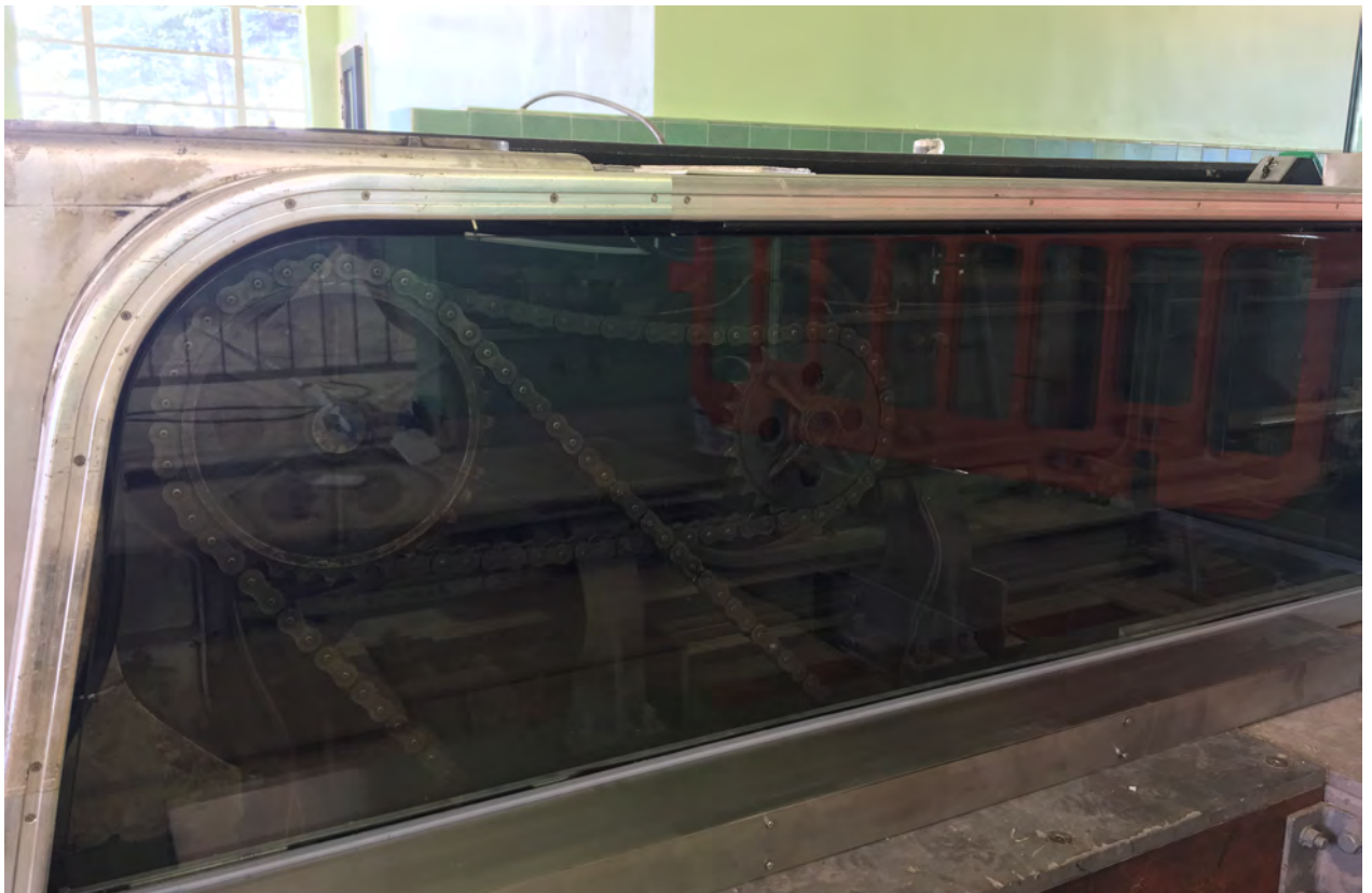
A glazed screen has been erected at the top and bottom landings to reveal the mechanical workings and chains which once powered the escalators.
