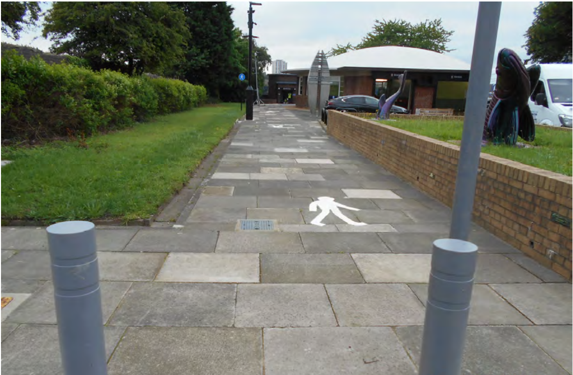
With the works at the tunnels substantially complete they were reopened to the public on the 7 August 2019.
