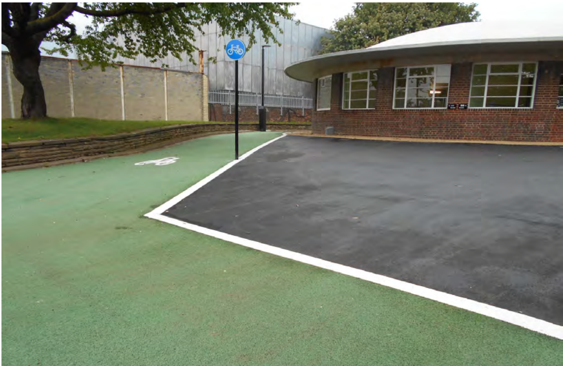
The landscaping and resurfacing works around the Howdon rotunda building guide cyclist to the vertical lift which provides easy access to the tunnels.
